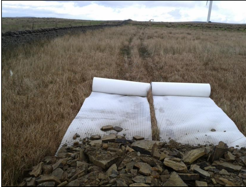
Plate 13: semi-permeable geotextile layer
