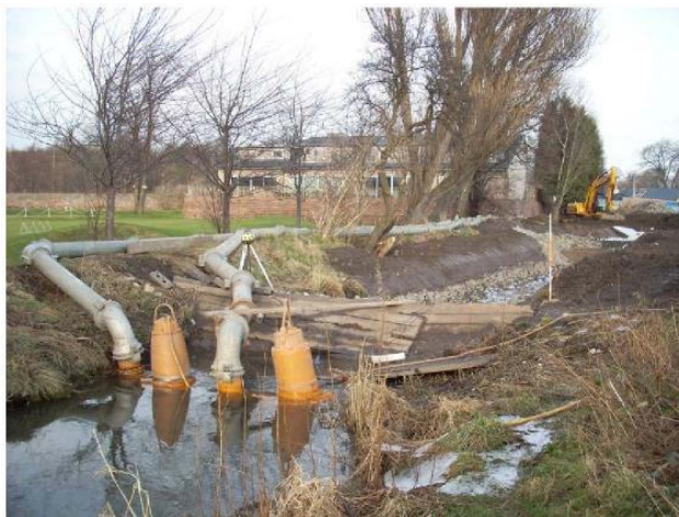
Plate 8: Full isolation – over pumping/siphon
