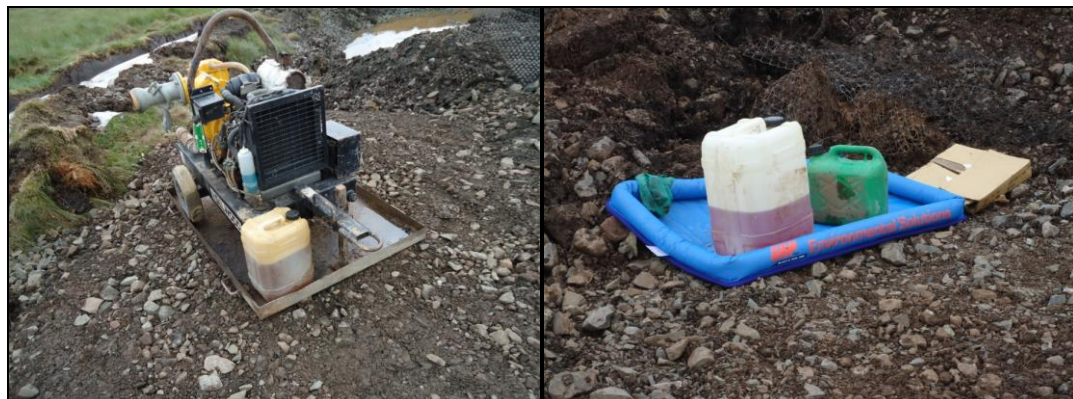
Plate 12: examples of drip trays and bunds
