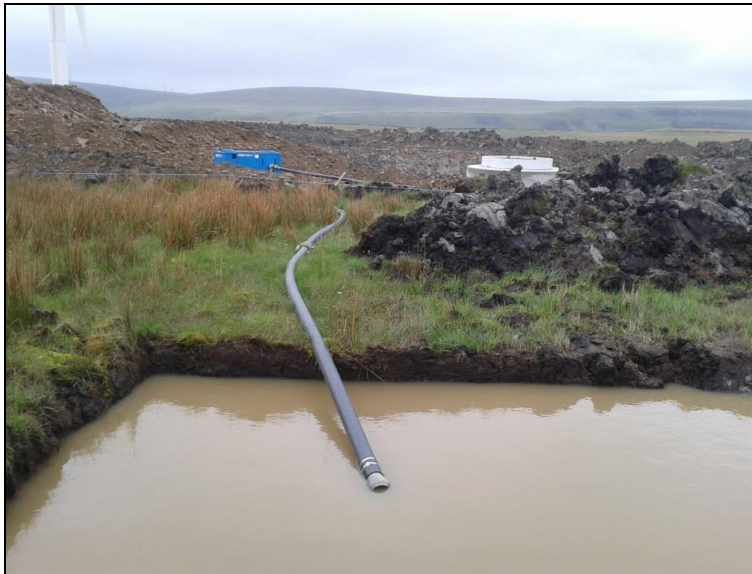
Plate 6: Typical 'Siltbuster' and settlement lagoon
